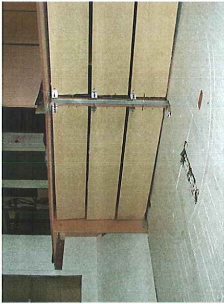
Figure 12-2 Vanes fully closed
